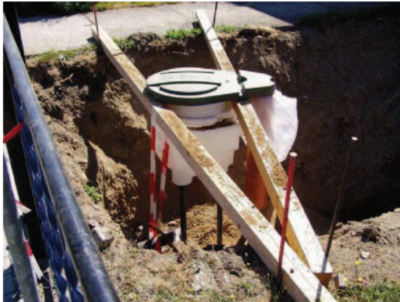
fig. 44 How to keep the G-Type collection chamber level during installation & backfill
